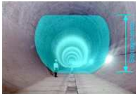
Inflow equalling up to 90% of the storage capacity of 240,000 m 3 (215,000 m 3 )
