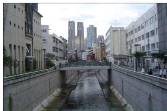
After the river channel was widened
