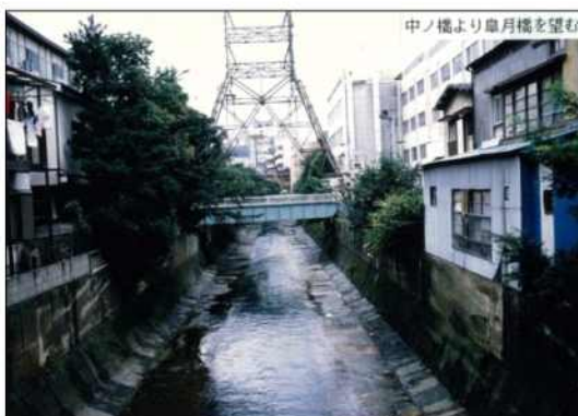
Before the river channel was widened
