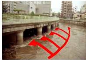
Inflow to the Kanda River intake facilities
